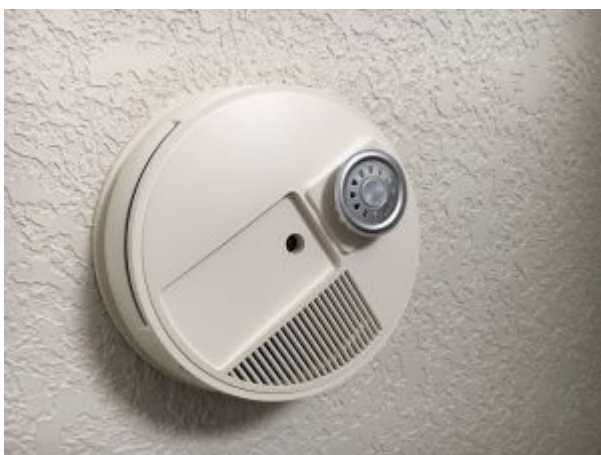
Testing Smoke Alarms
